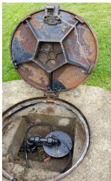
Figure 6: Borehole fully capped and sealed and in a locked chamber
