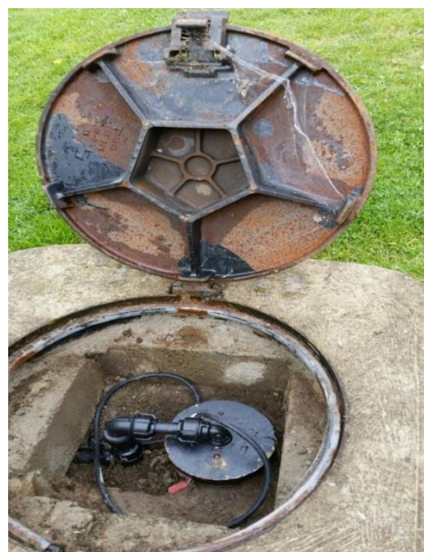
Figure 6: Borehole fully capped and sealed and in a locked chamber
