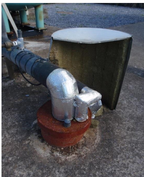
Figure 5: Wellhead constructed above ground level and borehole fully capped and sealed
