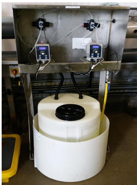
Figure 7: Sodium Hypochlorite disinfection system with bunded day tank and duty and standby dosing pumps
