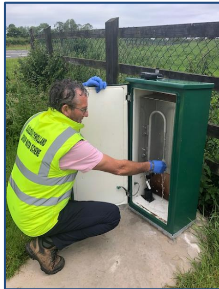
Figure 2: Caretaker taking chlorine residual sample
